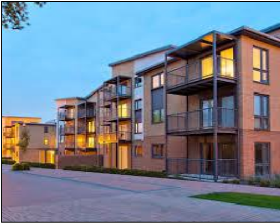
The Blocks at Night
